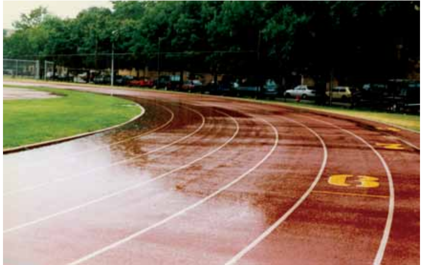
Running track without effective drainage
